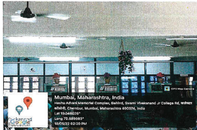
Wi-fi Router at Fifth Floor Library
